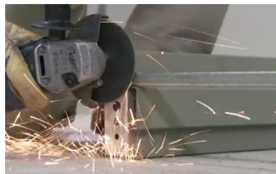
FIG. 8 – PROPERLY GRIND OFF SHIPPING BAR
