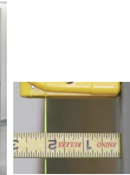
FIG. 14 – MASON SHOULD CHECK PLUMB, LEVEL, SQUARE BEFORE BEGINNING
