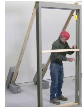
FIG. 14 – MASON SHOULD CHECK PLUMB, LEVEL, SQUARE BEFORE BEGINNING
