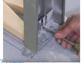
FIG. 11 – TEMPORARILY BRACE FRAME
