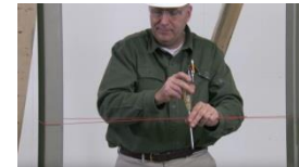
FIG. 14 – MASON SHOULD CHECK PLUMB, LEVEL, SQUARE BEFORE BEGINNING
