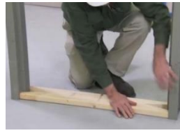
FIG. 11 – TEMPORARILY BRACE FRAME
