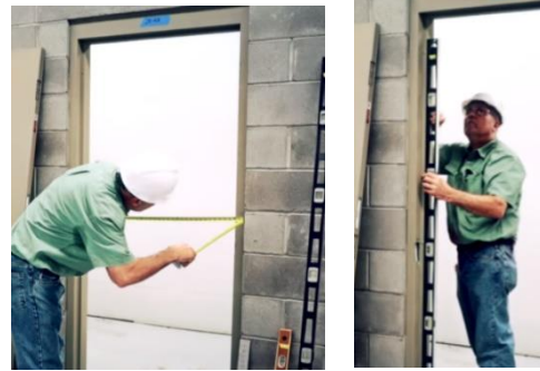
FIG. 23 – CHECK PLUMB, LEVEL AND SQUARE PRIOR TO DOOR INSTALLATION
