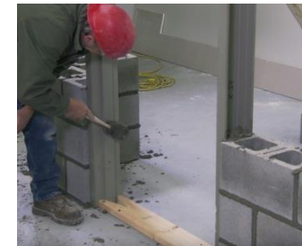
FIG 15. LAY BLOCK, CHECKING FOR PLUMB, LEVEL AND SQUARE EVERY TIME YOU MAKE AN ADJUSTMENT
