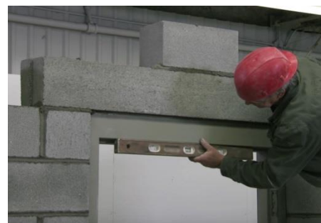
FIG. 19 – TYP A HIGH PSI PREFAB CONCRETE LINTEL IS USED, ALTHOUGH PROPER STEEL LINTELS MAY ALSO BE SPECIFIED. REF NON-TORNADO SDI/ALLEGION MASONRY INSTALL VIDEO min 7:50-8:30. ENSURE NO SAGGING.
