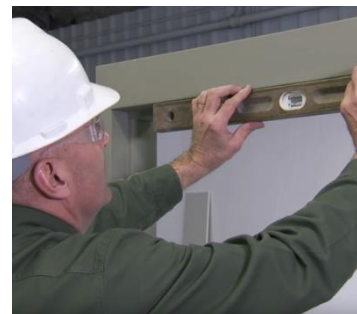
FIG. 18 – MASON CHECKS PLUMB, LEVEL, SQUARE BEFORE LAYING BLOCK AND THROUGH BUILD PROCESS
